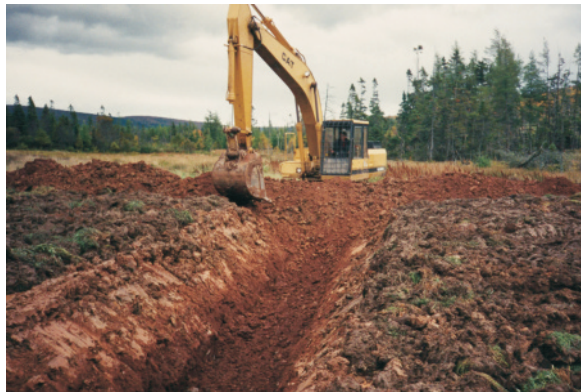
Figure 6. Deep and shallow zones of wetland with berm constructed from subsoil.
