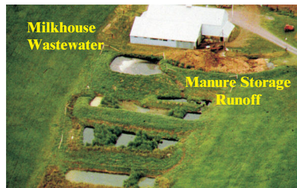
Figure 5. Aerial photo of constructed wetland in Pictou County, Nova Scotia on a 5% slope using a terrace type system.
