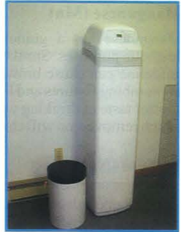
Oxidation Filtration System Used to Remove Iron, Manganese and Hydrogen Sulfide
