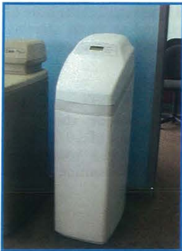
Water Softener Used to Treat Hard Water by Removing High Levels of Calcium and Magnesium
