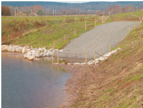
Figure 1. A newly prepared limited access ramp.
