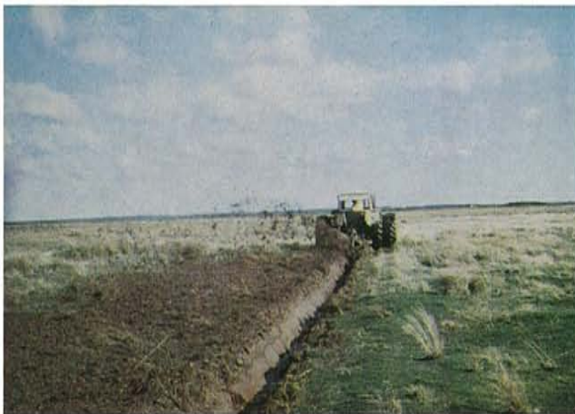
Figure 15. A Rotary Ditcher Excavating a Shallow Open Ditch on Dykeland.
