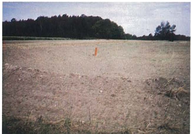
Figure 22. Surface Inlet Riser Pipe Installed in a Surface Water Collection Area.
