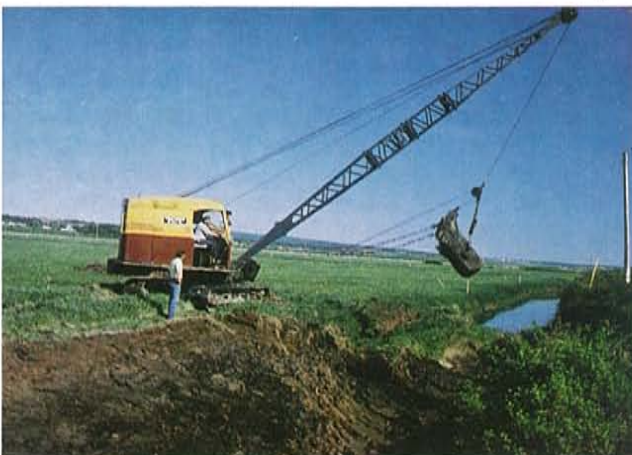
Figure 12. A Dragline Excavating a Large Open Ditch.
