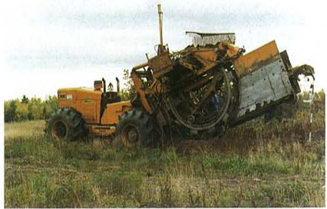
Figure 16. A Subsurface Drainage Trencher Preparing to Install Drainage Tubing.
