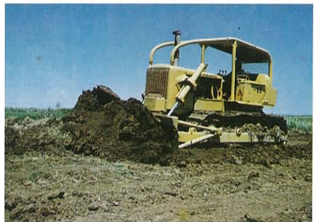
Figure 14. Dykeland Forming Using a Crawler Tractor.
