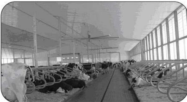
These fan units may be up to 7.2 m (24 ft) in diameter and are operated by a 1–2-hp motor. While the units are expensive to purchase, the payback period falls into the 4–5-year range, depending on the electricity prices and installation costs at the time.
