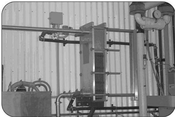
The most common type of pre-cooler consists of a series of stainless steel plates separated by gaskets that form flow channels on opposite sides of each plate. Cool well water flows down the channel on one side, while warm milk flows up the other side. The milk's temperature drops as it transfers its heat to the cool water on the opposite side of the plate. The plate heat exchanger is extremely efficient for fast pre-cooling.
